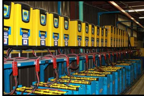
When positioning battery charger cabinets, consideration should be given to the charger DC cable lead length. It is important to design the battery charger layout in a manner that enables the charger DC cable leads to connect to the battery, yet ensures that the charger manufacturer DC cable lead length specification is not exceeded.
