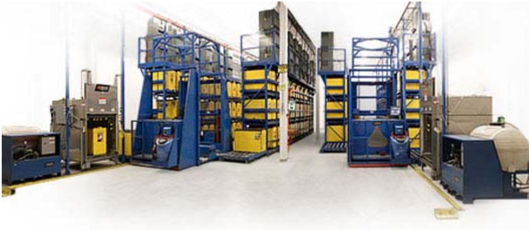
The battery room must have adequate electrical service and should be located near a main power feed, as distance from the power feed will increase costs. Chargers, ventilation, heating, cooling, and battery handling equipment all require electricity and should be considered when calculating the power requirements for the battery room. Plumbing, including drainage, will also be needed inside the battery room for battery filling and washing, as well as safety eye washes and showers.
